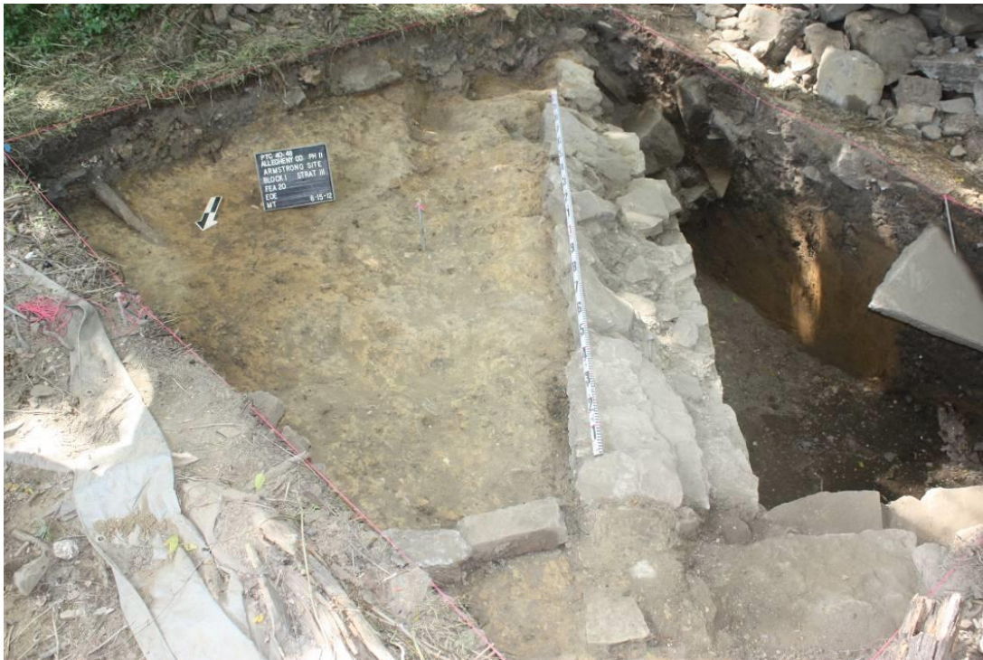
View of the clean fill layer exposed on the exterior of the house foundation.
